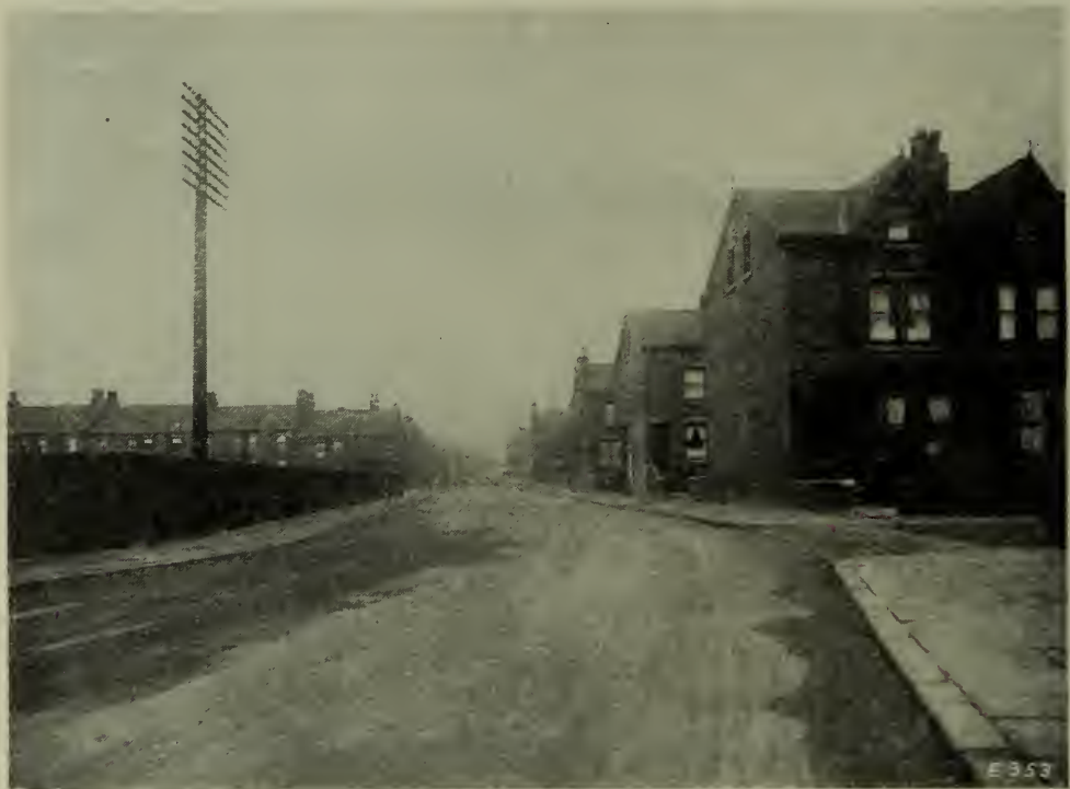
BURTON ROAD—AFTER COMPLETION.
